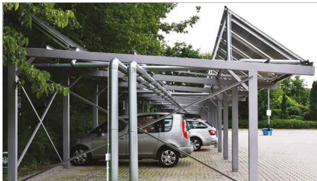
Supporting structure. Photovoltaic panels at Statistics Poland building
